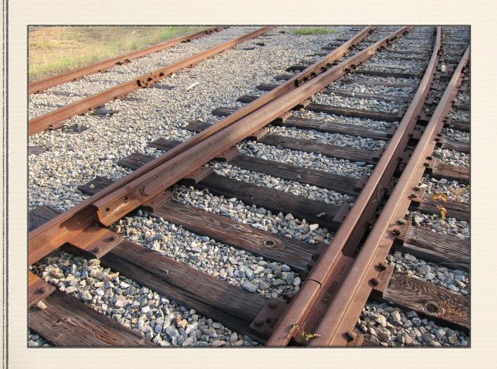
Ballasting is the loose stone placed between railroad ties to provide drainage and help keep the rails from shifting. It's the reason most track is raised a little bit above ground level.
